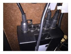
**Step 2** - Make sure that all cables to the black control box under the work surface are plugged in snugly (unplug and then plug back in).
