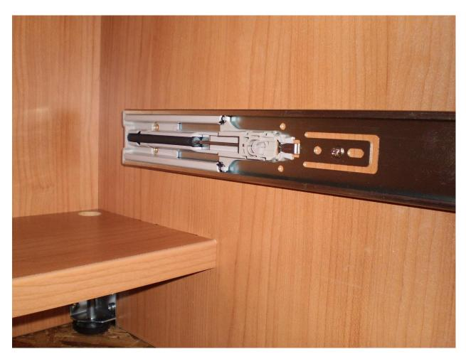
After the release lever is locked into place the Easy-Close drawer slide is ready for the drawer box to be placed back into the cabinet.
